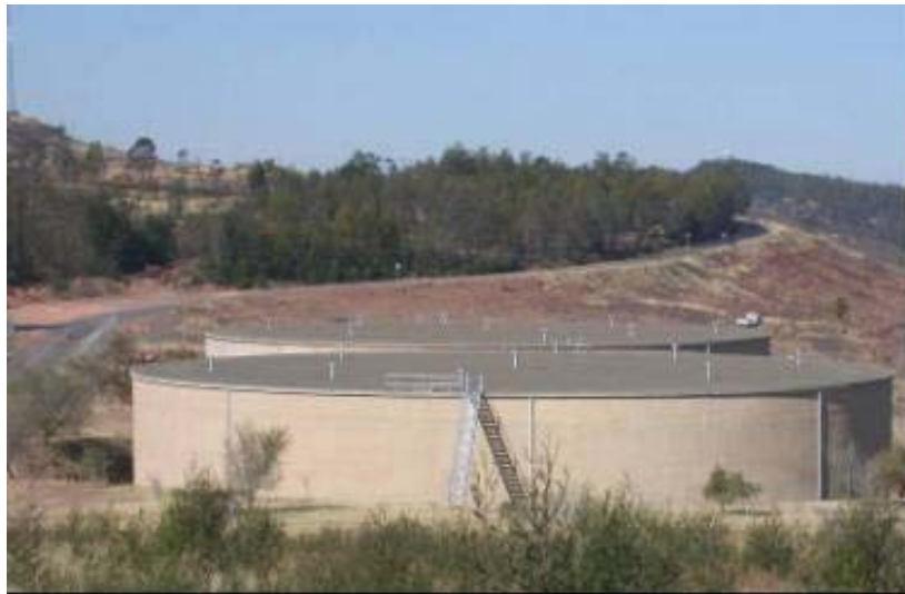
Figure 7: Concrete Water Reservoir
