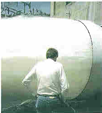
A Hartman Model 117 Fixed Cone Valve with hood provides containment of the jet, while discharging 1100 cfs.
