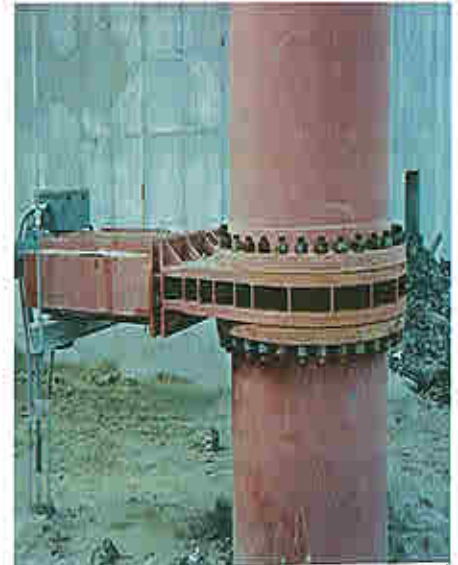
16" and 20" Flexgate Valves at the Clariton, PA WWTP
