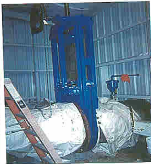
30" Flexgate Valve in Lithia, FL.
