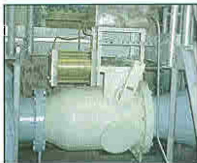
Model 711 Axial Flow Sleeve Valve with pilot control
