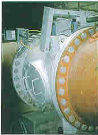
Model 711 Axial Flow Sleeve Valve
