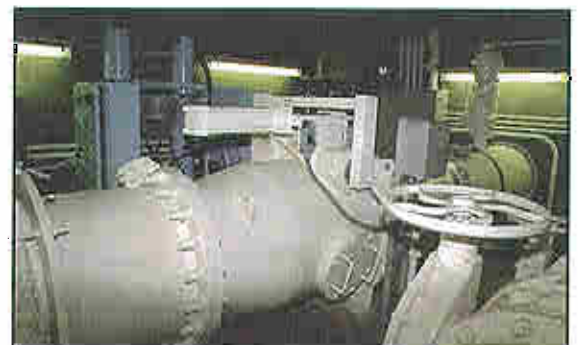
This Model 711 Axial Flow Sleeve Valve has a 24 inch inlet and outlet with a 20 inch sleeve.
